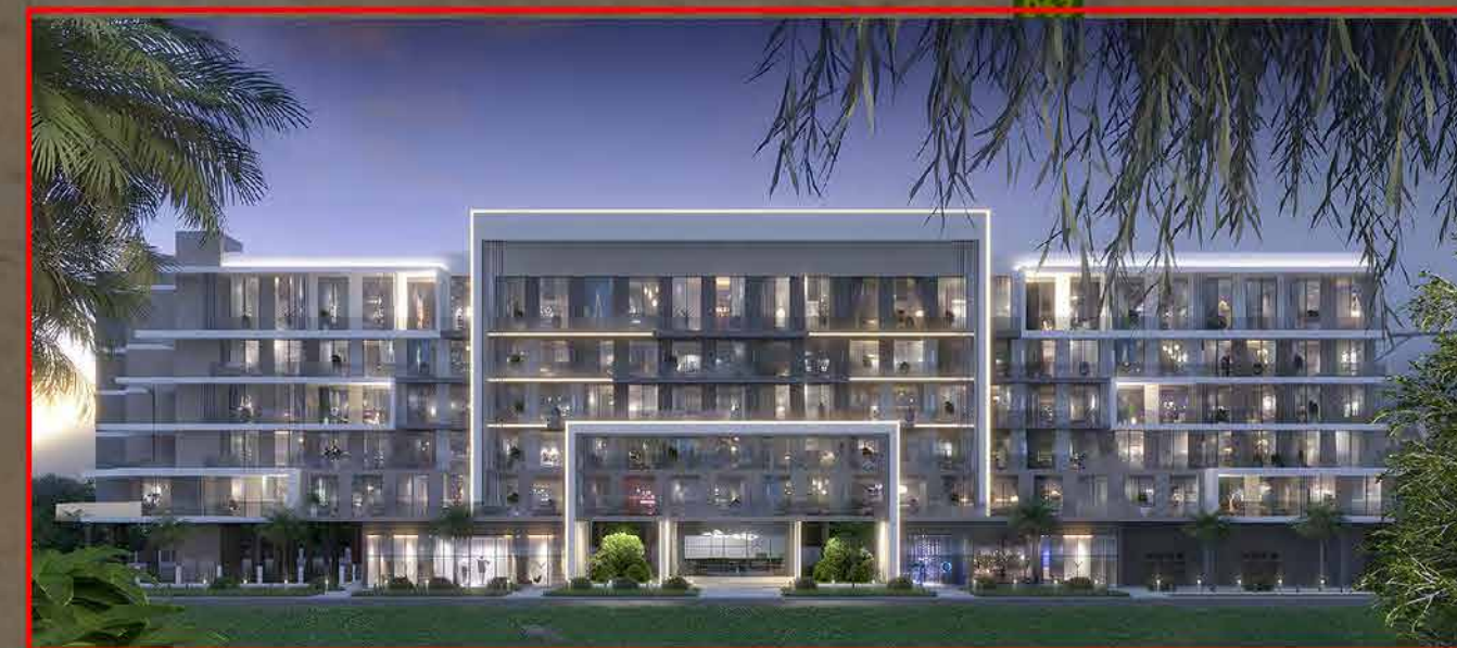
LAYA COURTYARD DUBAI STUDIO CITY, UAE
